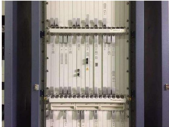
Gambar 1.14 *Serving GPRS Support Node (SGSN)*
