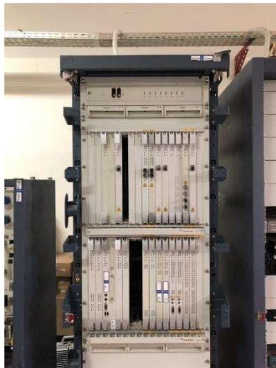
Gambar 1.9 *Radio Network Controller (RNC)*
